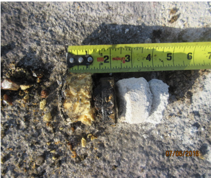
3. ROOF CORE ON AREA "D"
