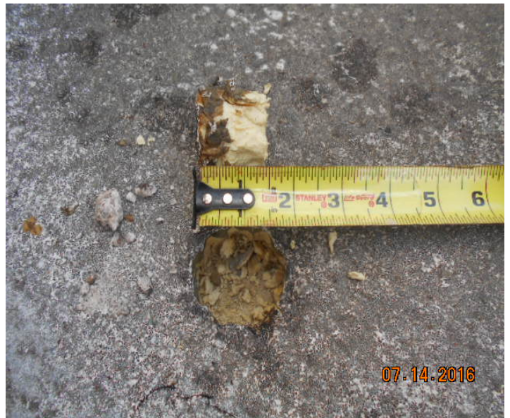
4. ROOF CORE ON AREA "H"
