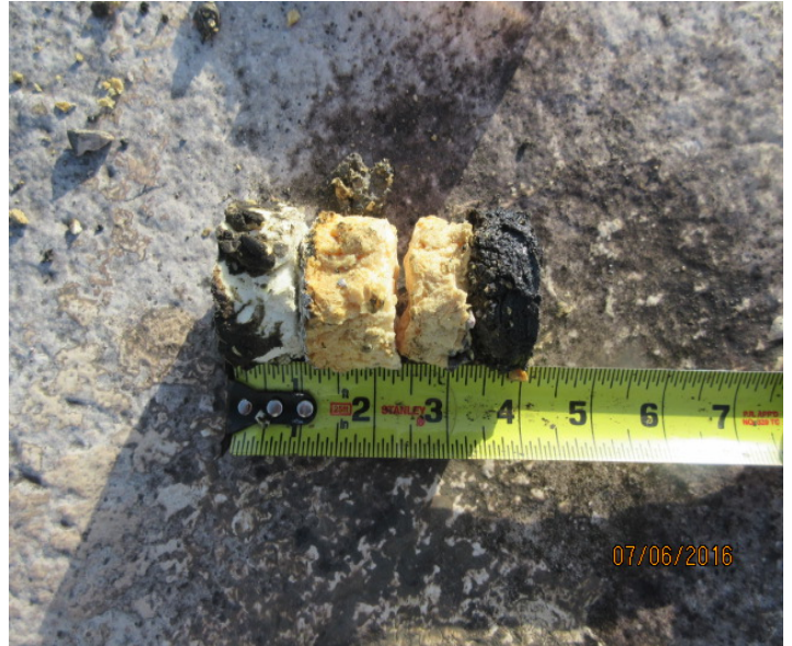
2. ROOF CORE ON AREA "B"
