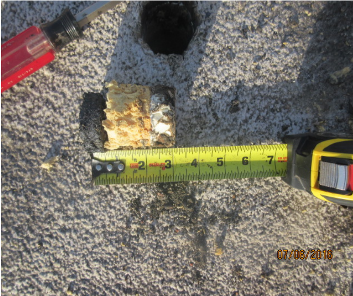
1. ROOF CORE ON AREA "A"
